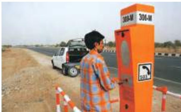
Fig. 7.10 : Emergency call box on NH-48
