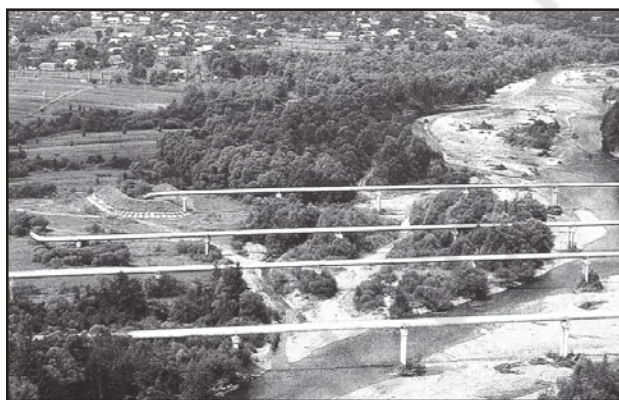
Fig. 7.17: Pipelines transporting natural gas in Ukraine
